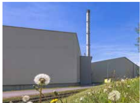
Fig.: Exhaust chimney for heat treatment plant 1
