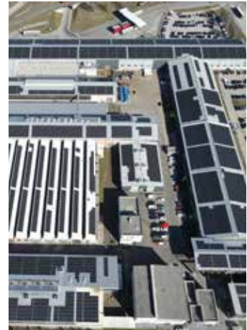
Fig.: PV plant in the coupling shop area
