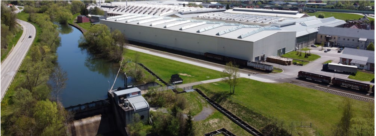
Fig.: Mürz hydropower power plant in Aumühl
