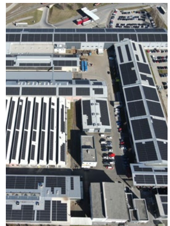
Fig.: PV system in the coupling shop area
