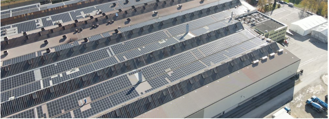
Fig.: PV system on the roof of the seamless tube rolling mill
