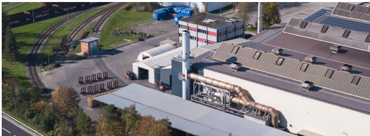
Fig.: Rotary Hearth Furnace exhaust stack with heat recovery
