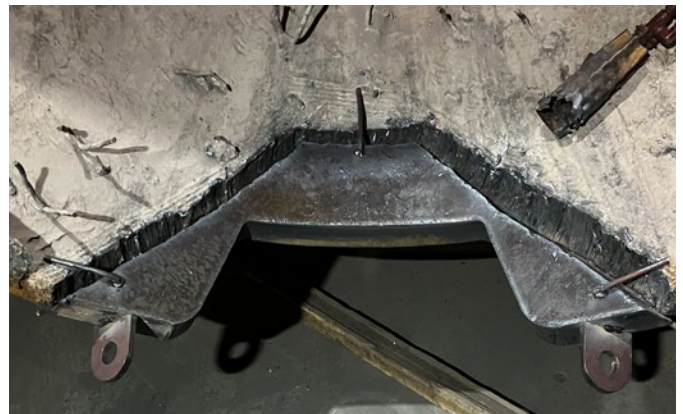
Figure 5: Pouring lip replacement in progress.
