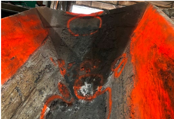
Figure 6: The interior view of a worn chute from a nickel smelter.
