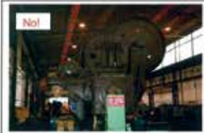
Figure 4.8a: Unprotected belt and wheels – beyond 2.5 m height it is dangerous for employees in direct way, but above 2.5 m e.g. the chain or hook of crane can be caught and a catastrophe initiated...
