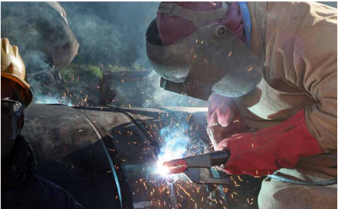
Pipeline Project: Südschiene, Austria 2010 Böhler FOX CEL 80-P
